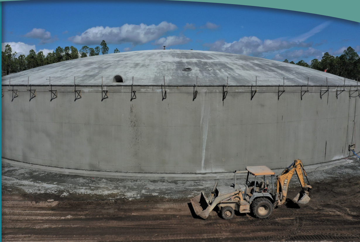
Watersound Water Storage Tank
